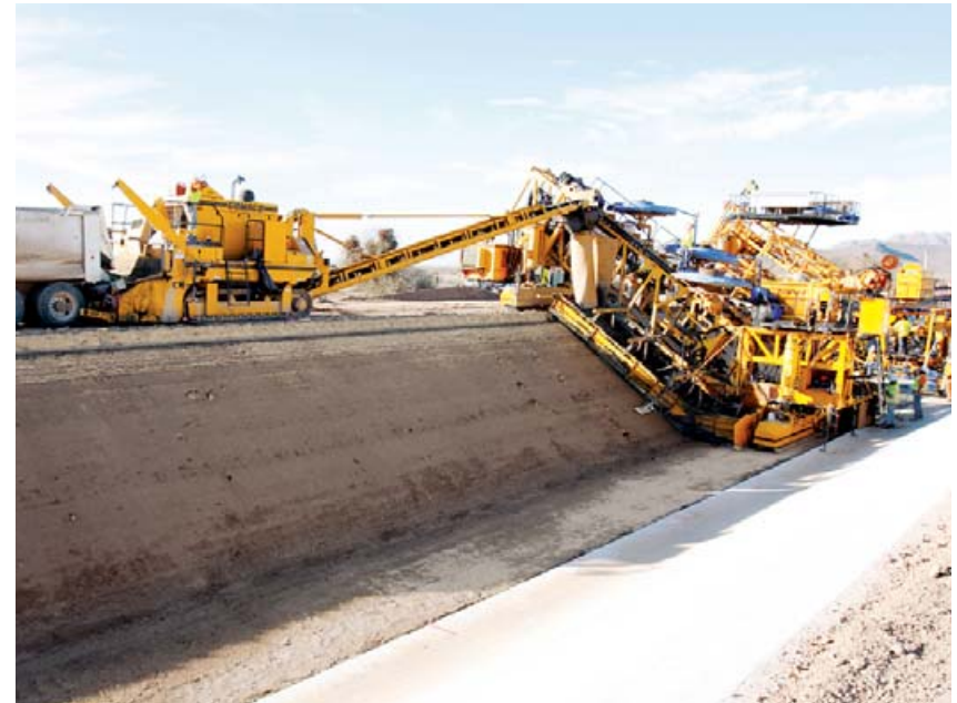
A GOMACO 9500 places the concrete for the canal paver.
