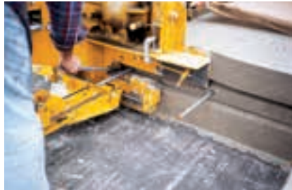
Female keyway with hydraulic side bar insertion (SBI) and vibration to the bar.
