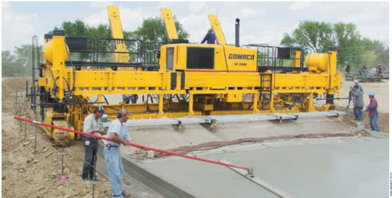
The two-track GP-2600 is slipforming a cul-de-sac with a 95 foot (29 m) inside radius. This machine is equipped with three frame-mounted bar inserters. This street in Wayne, Nebraska, is being slipformed full width with integral curb on both sides.
