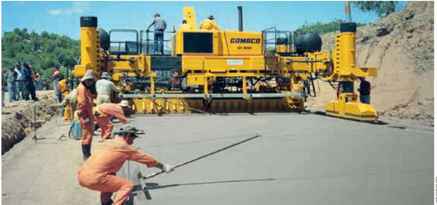
This versatile four-track GP-2600 slipforms a 24 foot (7.32 m) wide concrete roadway near Cochabamba, Bolivia.
