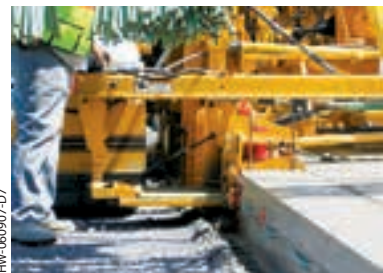
Trailing form with air-powered bar insertion.
