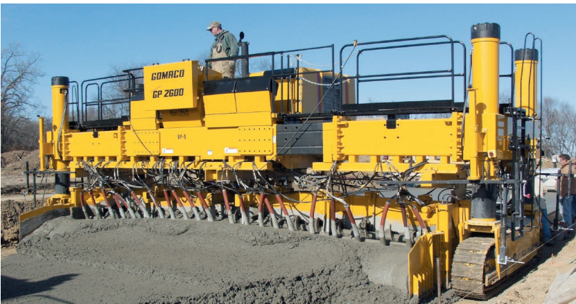
Hydraulically pressure-compensated sideplates provide edge control and consistent depth.
