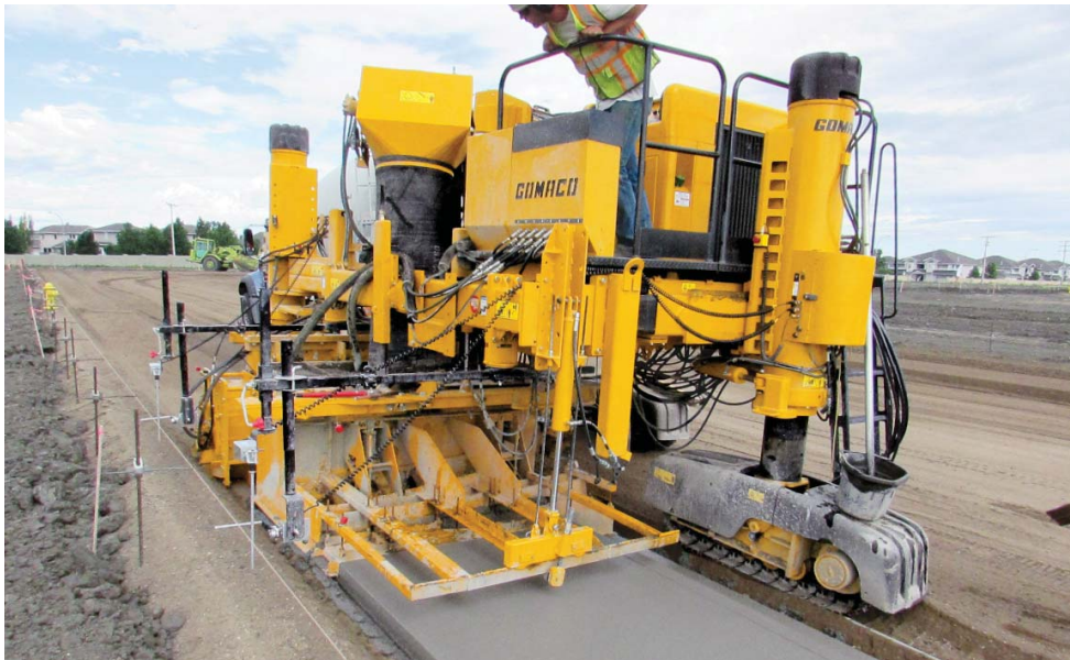
Five foot (1.52 m) wide monolithic sidewalk is just one application the Commander III can slipform with ease.
