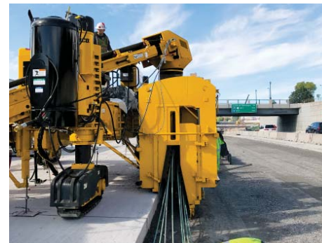
A front view of the continuous steel being fed into the machine.
