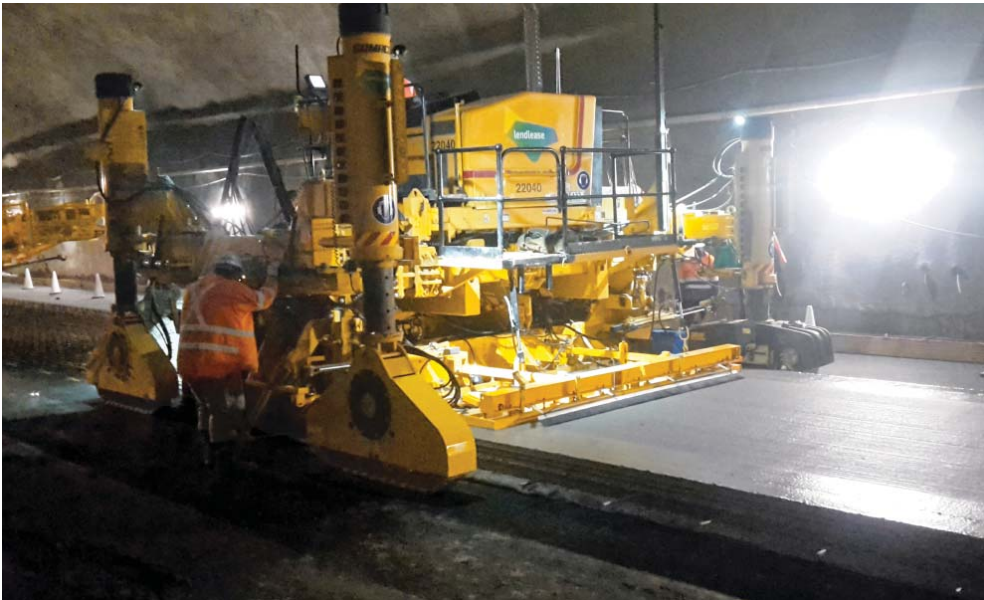
The GOMACO four-track Commander III with 3D machine guidance slipforms the floor of a tunnel at 14.7 feet (4.5 m) wide over continuous reinforced steel ahead of the paver. This Commander III is using high-rise tracks that are only six inches (150 mm) wide, for minimum clearance.
