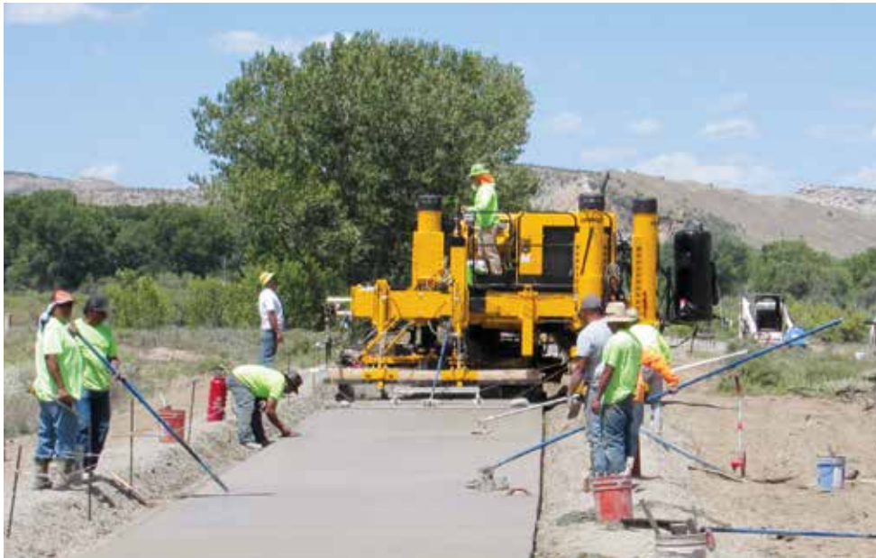
A ten foot (3.05 m) wide bike path is slipformed by the three-track Commander IIIx.
