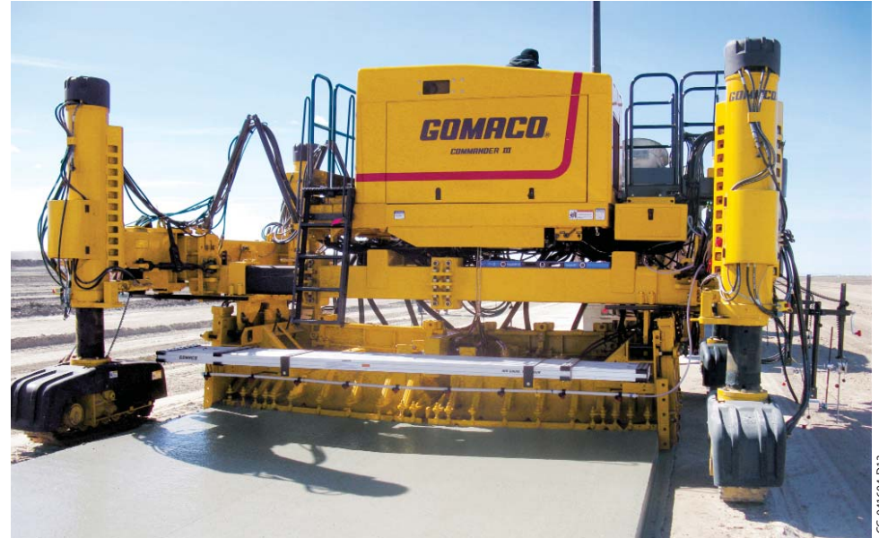
Equipped with a two inch (50.8 mm) inverted mold this Commander III four-track slipforms a 14 foot (4.27 m) wide slab on a dairy farm.
