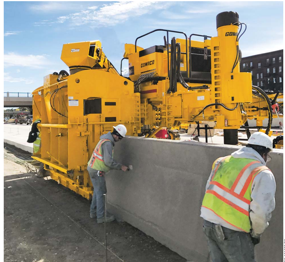
This barrier mold is mounted onto the four-track Commander III and is slipforming a 42 inch (1067 mm) tall variable barrier with continuous steel being fed into the mold. The Commander III is positioned in the transverse mode for barrier paving.
