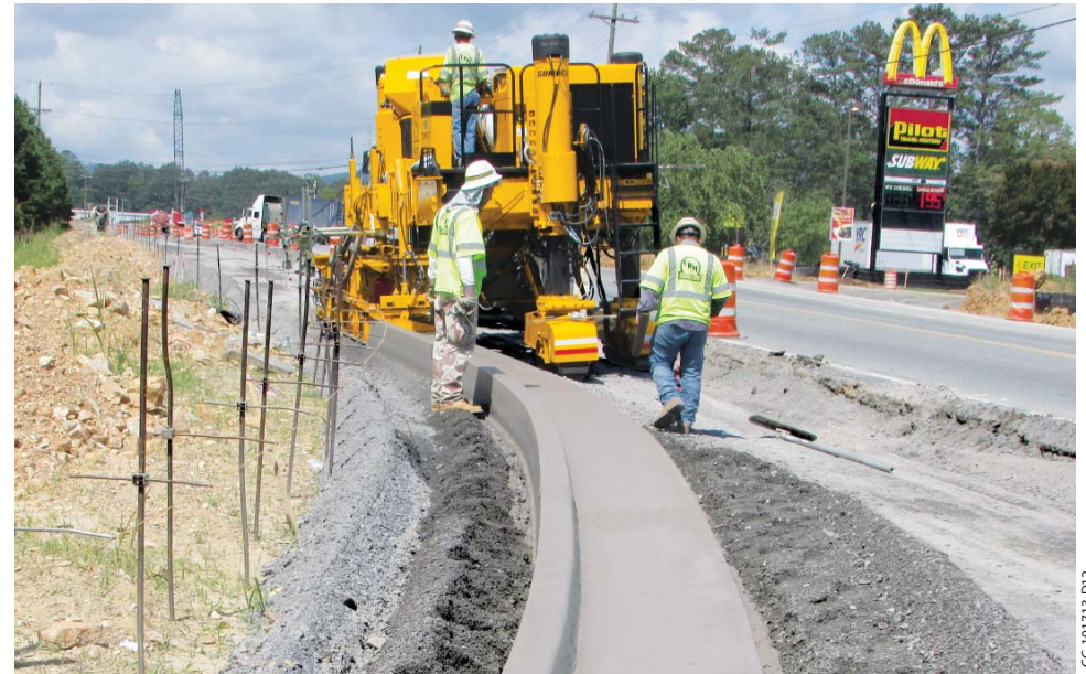
The Commander IIIx features a platform that has a skid-resistant surface on the walkway for safety and is vibration isolated for operator comfort during a full day of slipform paving.
