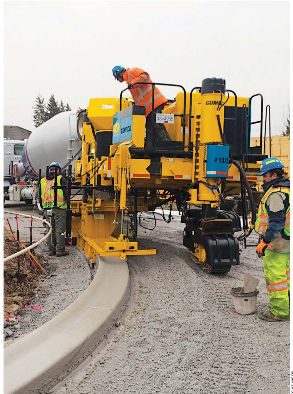
The three-track Commander III slipforms curb and gutter through a radius in a residential area. The trimmerhead sideshifts on-the-go throughout the radius.
