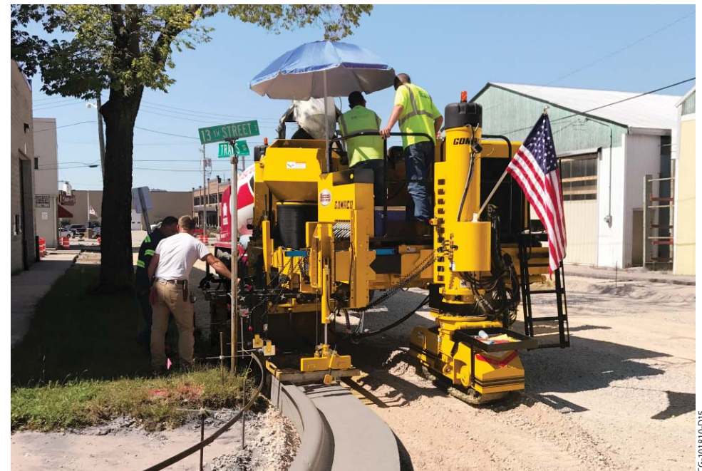
The three-track Commander IIIx slipforms curb and gutter in a residential area.
