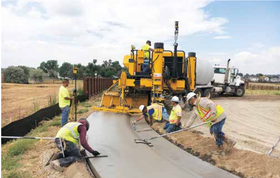
Using 3D machine guidance, the Commander IIIx slipforms monolithic sidewalk and curb and gutter within a new subdivision.
