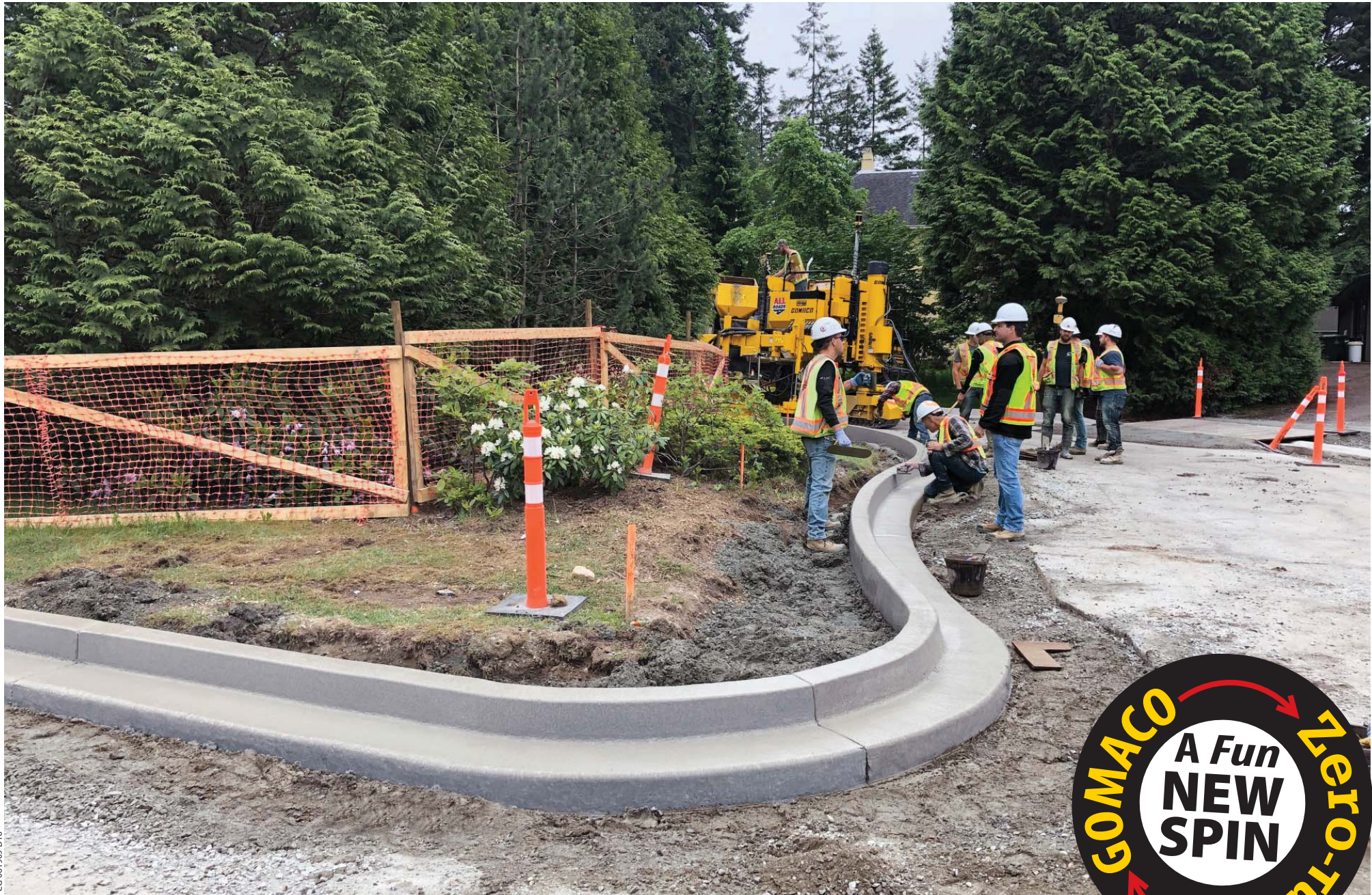
The GOMACO Commander IIIx, three-track, uses rotary-sensored slew drives on each track to slipform this curved curb and gutter on a residential street in Canada. This Commander IIIx is equipped with GOMACO Remote Diagnostics (GRD) to assist in fleet management through your cell phone or laptop computer.
