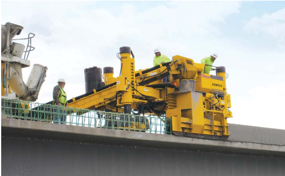
The GOMACO three-track Commander III slipforms parapet over steel on a bridge project.
