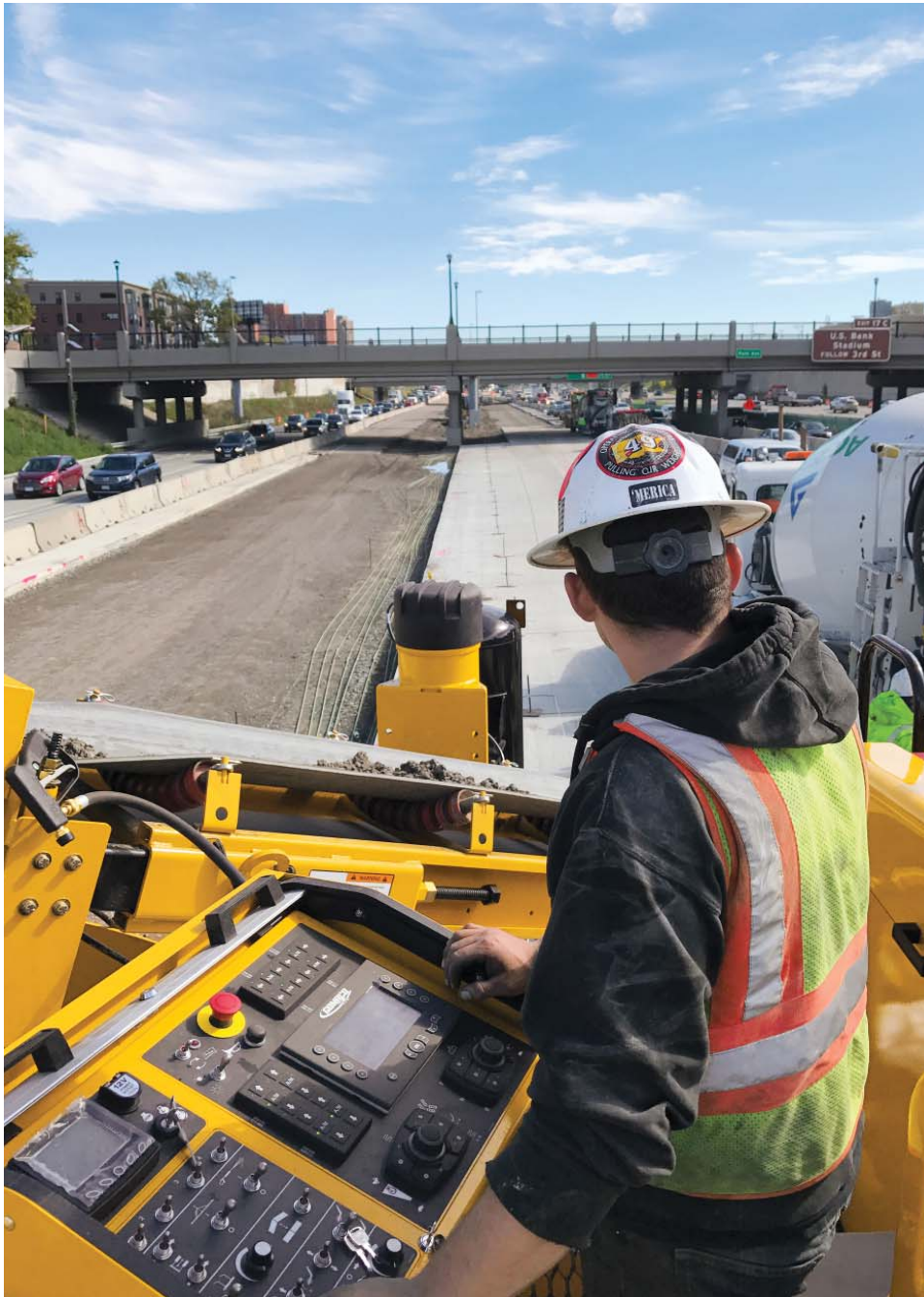
The operator has a complete view of the paving operation, from the delivery of concrete to the finished product, while always maintaining full control with the pivoting operator's panel.
