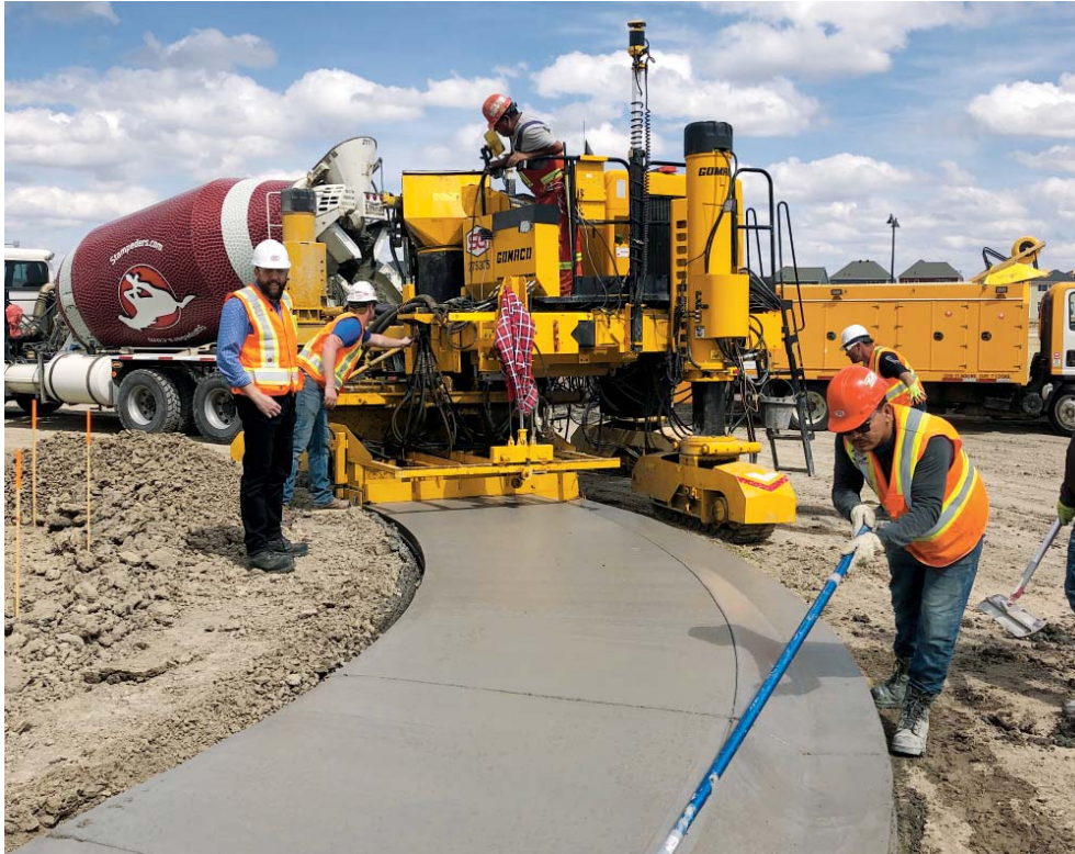
The three-track Commander IIIx slipforms monolithic sidewalk and curb and gutter.
