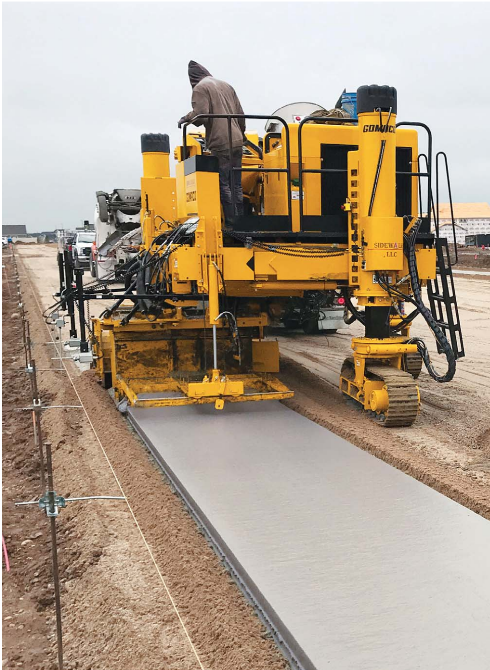
A five foot (1.52 m) wide sidewalk in a new housing development area is being slipformed by the Commander IIIx three-track using trim and pour for maximum material utilization.
