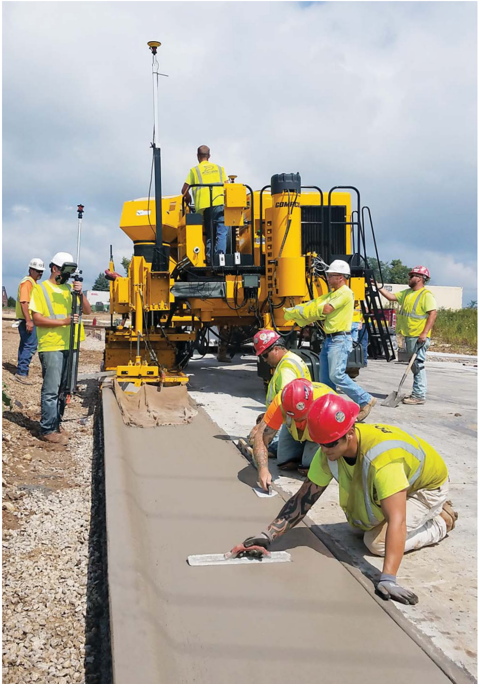
The three-track Commander III slipforms scab-on curb and gutter using 3D machine guidance for steering and grade.
