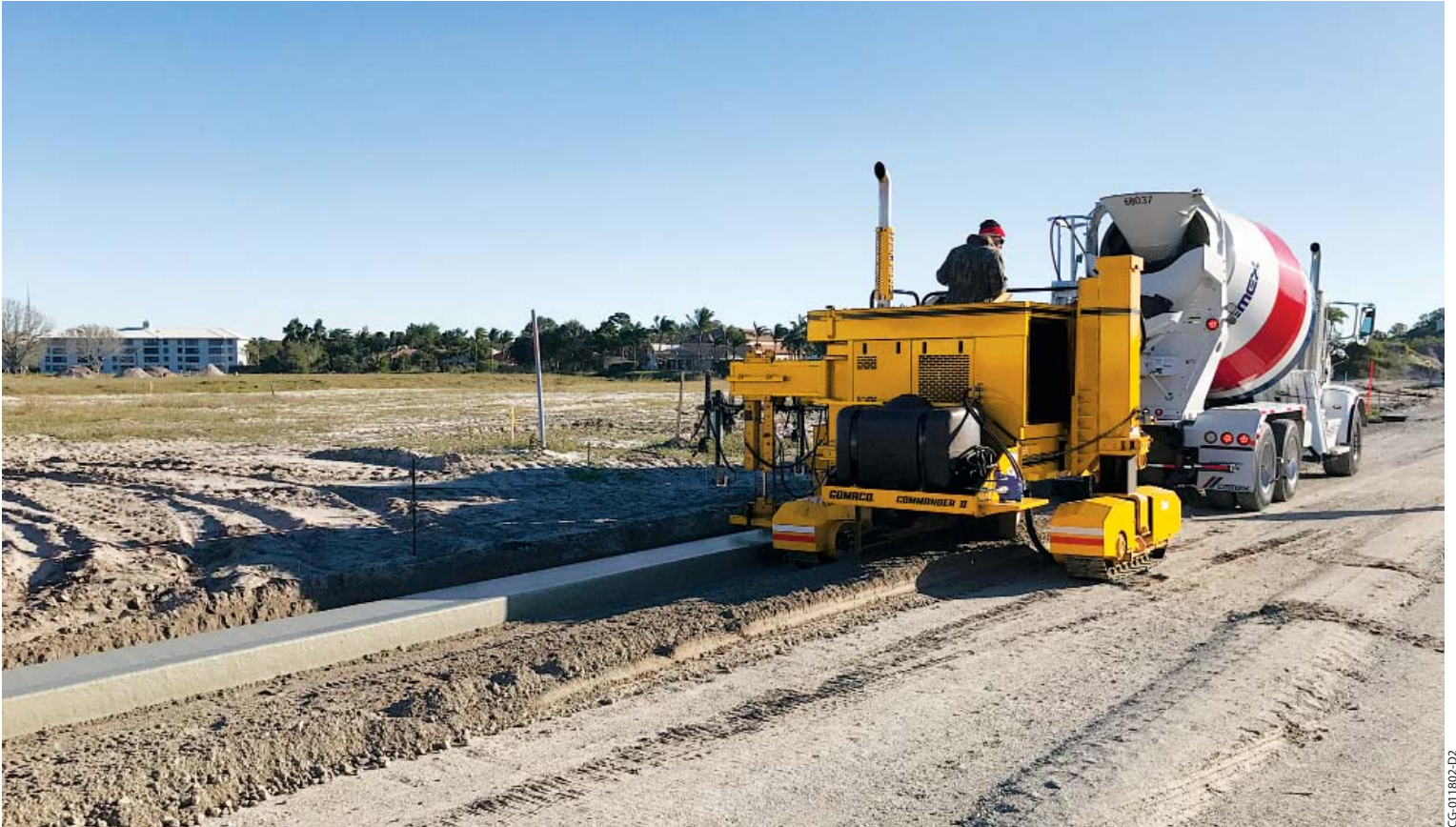
The GOMACO Commander II is able to slipform curb and gutter utilizing the smooth travel speeds of the G+ control software.
