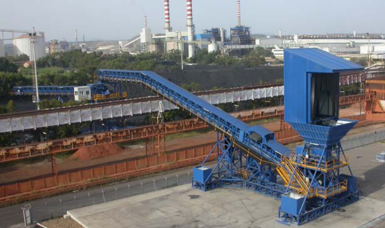
Cagliari, Italy: Coal handling system
