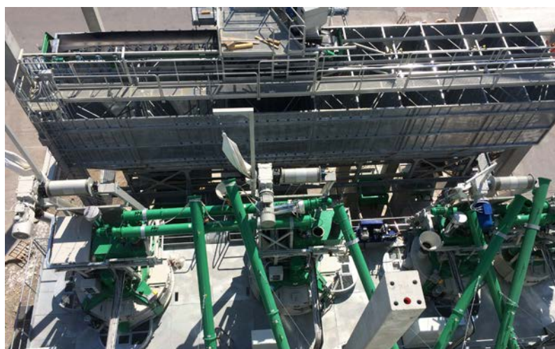
Bergamo, Italy: Pre-cast factory
